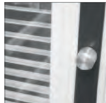
Blinds can be integrated in double glazed panels.
